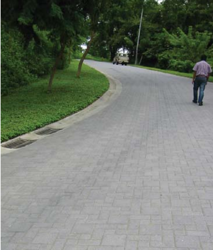
Figure 2. This Costa Rican road reaches up a mountain at maximum 25% slope. The paving pattern imitates a herringbone which is recommended for sloped applications. This photo shows a four year-old pavement.
