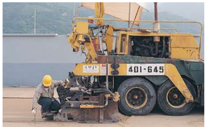
Figure 6. Mechanical screeding is the most efficient method of bedding sand installation. In the largest projects, a laser guided asphalt spreader (right) can be used to accurately screed bedding sand.
