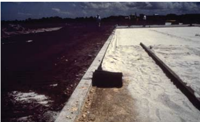
Figure 8. Woven geotextile contain bedding sand from migrating into curb joints or between the curb and base.
