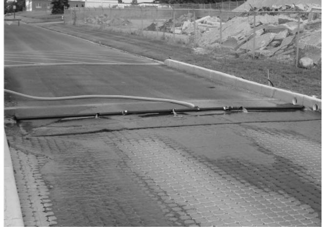
**Fig. 1.** Currie Barracks permeable pavement installations with field application device shown in right figure (UNI Eco-Stone in foreground, porous asphalt in background).
