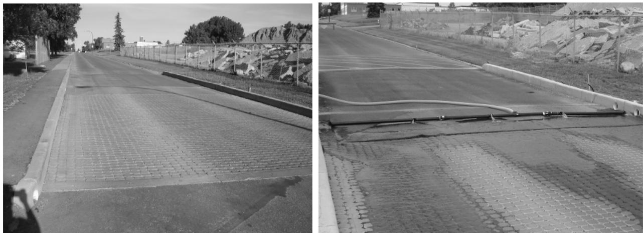
**Fig. 1.** Currie Barracks permeable pavement installations with field application device shown in right figure (UNI Eco-Stone in foreground, porous asphalt in background).
