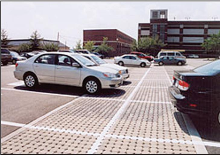
*Figure 2.3.5a Reduced Parking Stalls with Permeable Paving Strips*
