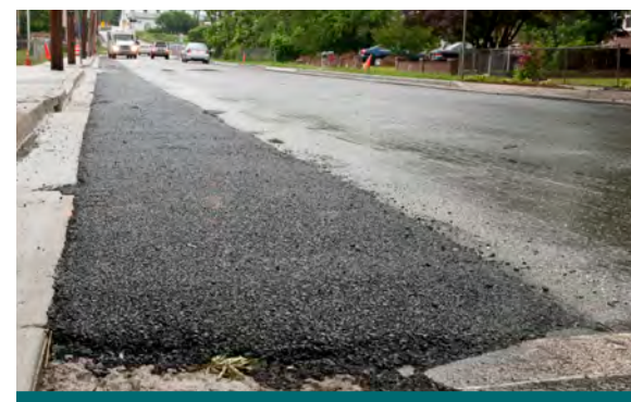
Figure 2.5.2: Porous asphalt was used to create a permeable bike lane in Edmondston, MD. As pervious asphalt can look quite similar to traditional asphalt, municipalities should track the location of permeable infrastructure to ensure that it is not re-paved in future roadwork. (Source: CVC)
