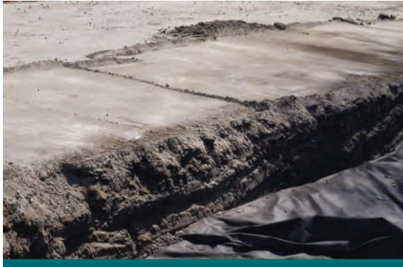
Figure 9.5.1: Sediment and dust accumulate quickly on a construction site. Daily cleanup and street sweeping were worked into the schedule at the Lakeview Project. (Source: Aquafor Beech)
