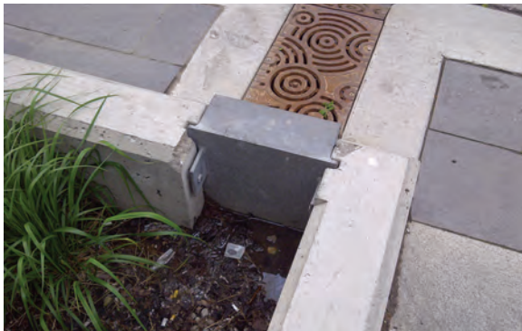
Figure 6.4.3: The gates on this bioretention planter in Kitchener, Ontario are designed to close during the winter season to prevent infiltration of chloride from deicing practices. (Source: Aquafor Beech)
