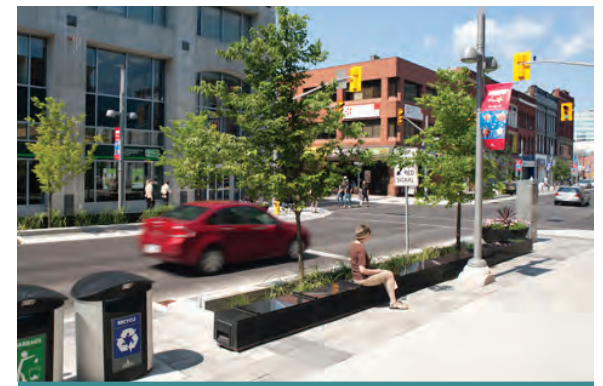
Figure 1.3.2: Bioretention planters are an integral part of Kitchener's new King Street streetscape. They not only help manage stormwater runoff from the road, but they also provide amenity value through street greening and providing pedestrians with a gathering space. (Source: City of Kitchener)
