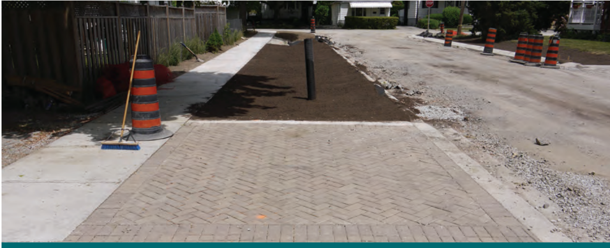
Figure 9.3.1: Construction activities including excavation, sawing, and delivery of materials can cause debris and sediment deposition across a construction site even during good weather. It is essential that bioretention soil media is not delivered and installed until the surrounding area is clean. (Source: Aquafor Beech)
