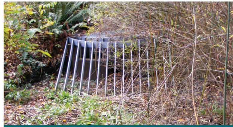
Figure 6.4.10: Overflow grate inverts should be surveyed to confirm that they will function as intended during infrequent storm events. Vegetation should be managed around overflow grate inverts to prevent clogging. (Source: Aquafor Beech)
