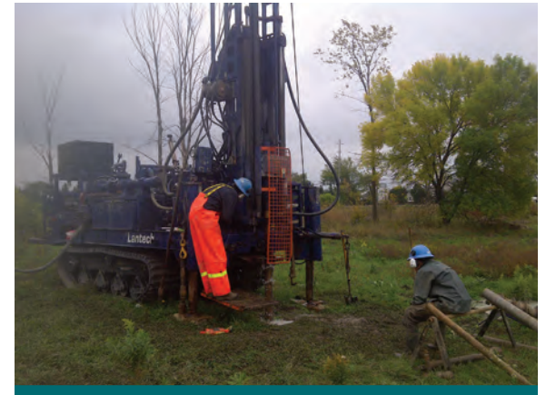
Figure 5.2.1: Before undertaking a geotechnical investigation, consider what equipment will be required. Where large equipment such as a drill rigs is required it is essential to ensure there is a safe ingress and egress for all equipment and people. Also consider how the work will affect user of the ROW and adjacent properties. Traffic controls may be required on confined or busy roads. (Source: Aquafor Beech)
