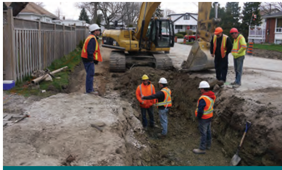
Figure 9.2.3: During the construction of the Lakeview Project the bioswale trench alignment travelled off-centre due to over-excavation. The team lead used the passive approach since the excavation could not be reinstated and the error did not cause negative impacts to the design. (Source: Aquafor Beech)
