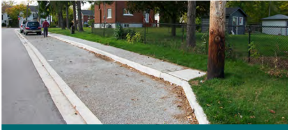
Figure 2.5.3: Pervious concrete requires a modified poring and setting approach when compared to standard concrete. Porous concrete was used to create a permeable parking lay-by in Streetsville in Mississauga. (Source: CVC)
