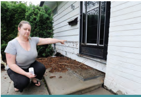
Figure 1.1.1: July 8, 2013 flooding also impacted private property. In this photograph a Mississauga resident shows the structural damage that took place to her home. (Source: Fred Loek, Mississauga News)
