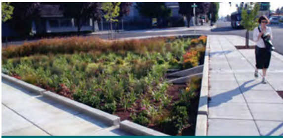
Figure 4.3.27: This large bioretention planter along an urban arterial replaced a large unused expanse of asphalt. (Source: Nevue Ingan Associates)
