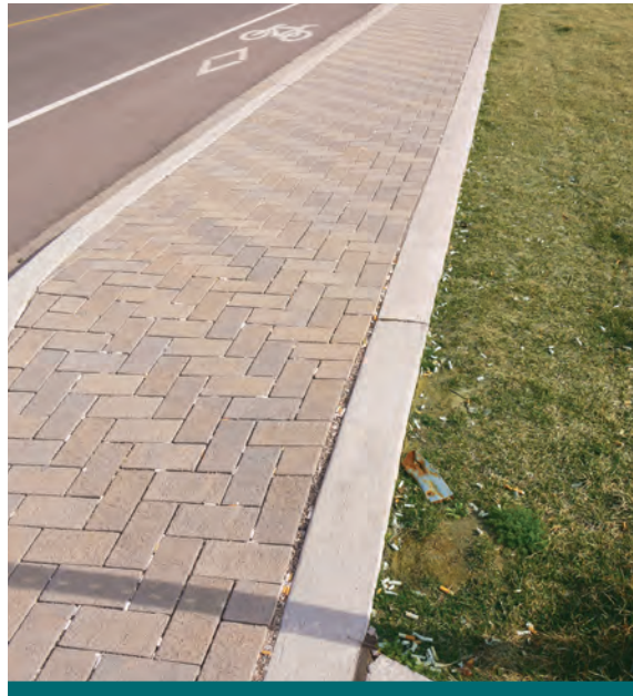
Figure 4.3.34: Further consideration of user behavior may have resulted in a different LID solution for this location. This section of sidewalk is a preferred smoking location for the adjacent business and the cigarette butt waste stuck between the permeable pavers will be an ongoing maintenance problem. (Source: CVC)
