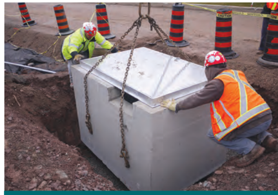
Figure 4.3.15: Prefabricated modules can be used on local industrial roads to capture high sediment loads. (Source: CVC)
