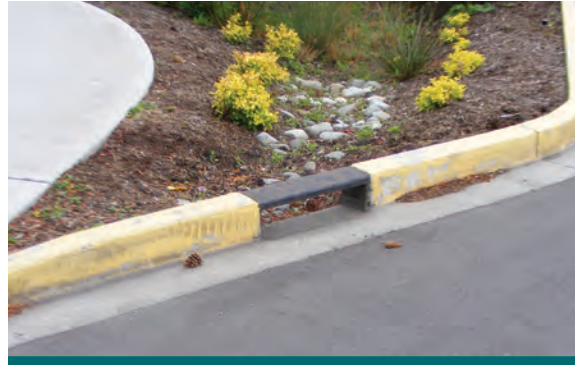
Figure 6.4.4: A covered curb cut can be used to provide the protection of a curb but allow runoff to enter the facility. (Source: Aquafor Beech)
