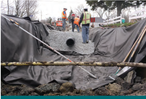
Figure 9.4.4: At the Lakeview Project a gas line was found to span the bioswale trench. Moving the gas line was not an option. An adaptive approach using avoidance was determined to be the best course of action. (Source: Aquafor Beech)
