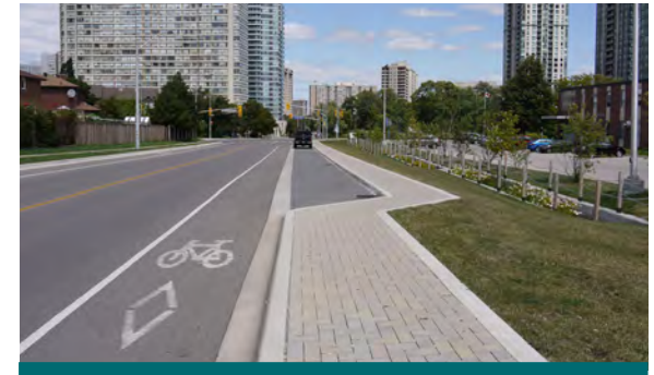
Figure 2.5.4: Permeable pavers can be used to create visual interest within the ROW. On Elm Drive, located in Mississauga, permeable pavers with different shapes and colours were used for parking lay-bys and the sidewalk. (Source: CVC)
