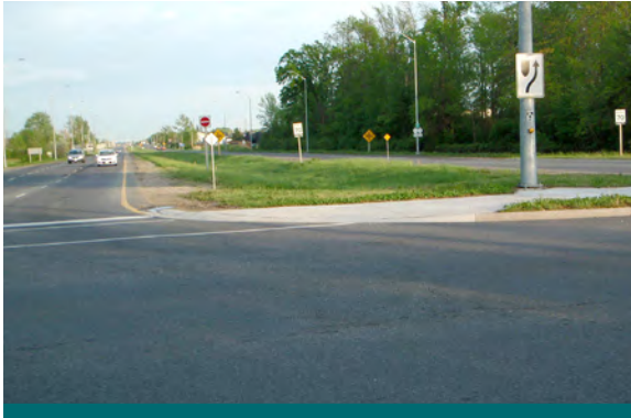
Figure 4.3.26: Major arterial road. (Source: Aquafor Beech)
