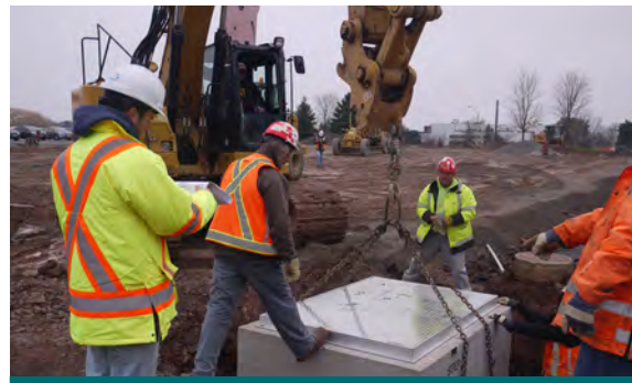
Figure 2.4.7: To maximize treatment and water balance benefits, proprietary stormwater treatment devices can be installed upstream of LID practices. (Source: CVC)
