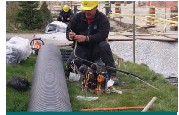
Figure 9.4.3: When utilities are damaged, expect additional people onsite. In this photo communications technicians establish service after damage to a cable at the Lakeview Project. (Source: Aquafor Beech)
