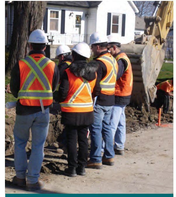
Figure 9.1.1: Team members on an LID construction site will include consultants, contractors, and municipal staff. It is essential that team members communicate and are aware of group and individual responsibilities. (Source: CVC)
