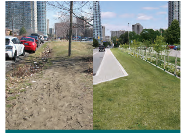
Figure 4.3.11: Before and after pictures of a residential collector, Elm Drive West in Mississauga, improved from a rural cross-section with degraded ditch to an urban cross-section with permeable paver parking laybys and sidewalk. The new design eliminated the degraded swales and improved safety for street parking. (Source: CVC)
