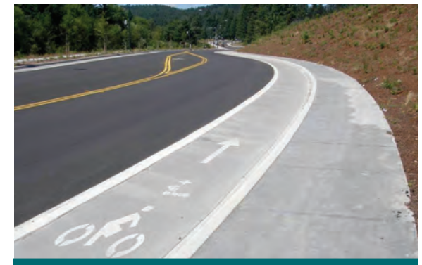
Figure 4.3.12: Pervious concrete bike lane and sidewalk in, City of Olympia, WA. (Source: City of Olympia)
