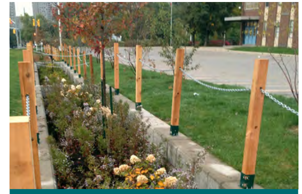
Figure 2.1.2: Bioretention planters aren't just for highly urbanized road ROWs. Planters were used to retain additional road runoff from Elm Drive in Mississauga. (Source: CVC)
