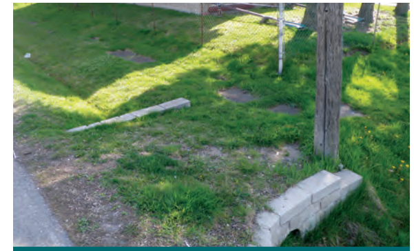
Figure 4.2.2: Unmaintained property access points that cross the conveyance path of the ROW may not be identifiable on background materials. (Source: Aquafor Beech)
