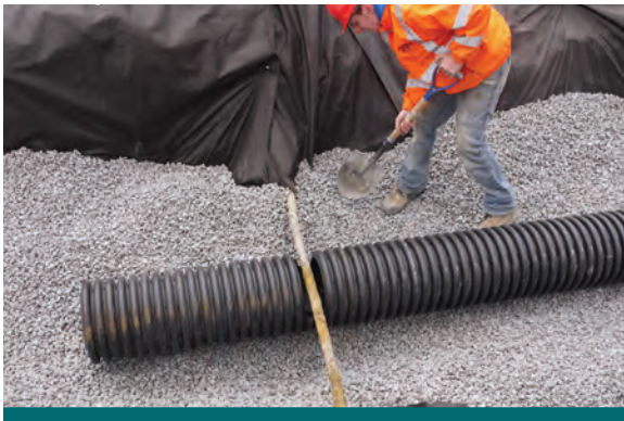
Figure 9.4.5: The above photo shows how the perforated pipe was installed around the exposed gas line at the Lakeview Project. A notch was cut in the perforated pipe and fit into place below the gas line. (Source: Aquafor Beech)
