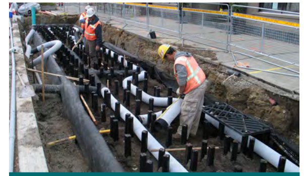
Figure 2.4.3: Installing the soil support system under the sidewalk on part of the Queensway in Toronto. (Source: Deep Root Inc.)
