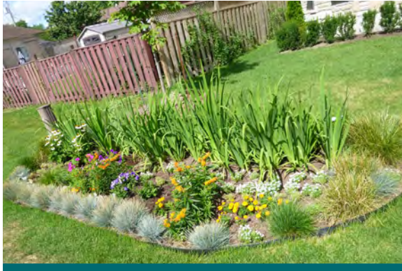
Figure 10.1.1: A photograph showing one the bioretention features in the Lakeview project maintained and even augmented with additional plantings by the homeowner. Private owner maintenance of boulevard bioretention units was found to be a practical approach for the Lakeview project, however, areas where there is a higher occurrence of renters the municipal or hybrid approach may be better suited. (Source: CVC)
