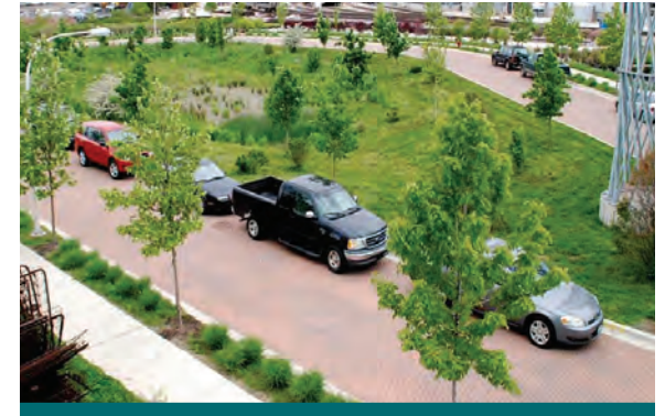
Figure 4.3.16: This light industrial and commercial road in Chicago uses permeable pavers from curb to curb and loops around a dry detention feature. (Source: ICPI)
