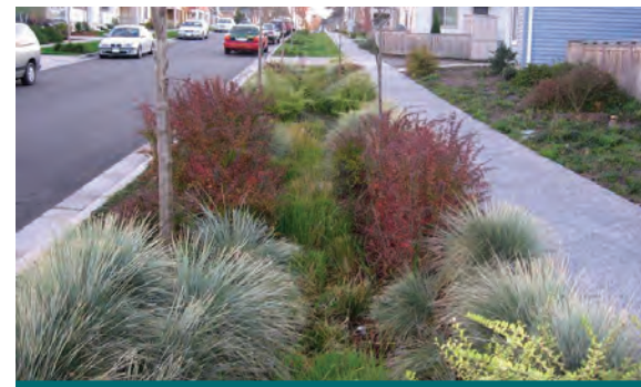
Figure 6.5.2: Boulevard bioretention projects are most successful on streets where residents own their homes and invest in their landscapes, such as in the image above. Note the year round interest, colour, and varied textures in the design above. (Source: CVC)
