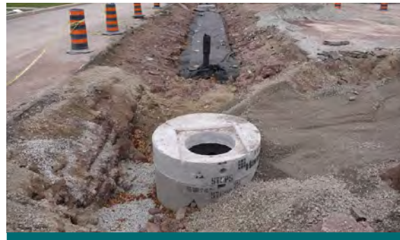
Figure 6.14.1: At the Elm Drive project, the design included a manhole for the collection of water quantity and quality samples, located downstream of the LID practices. (Source: CVC)
