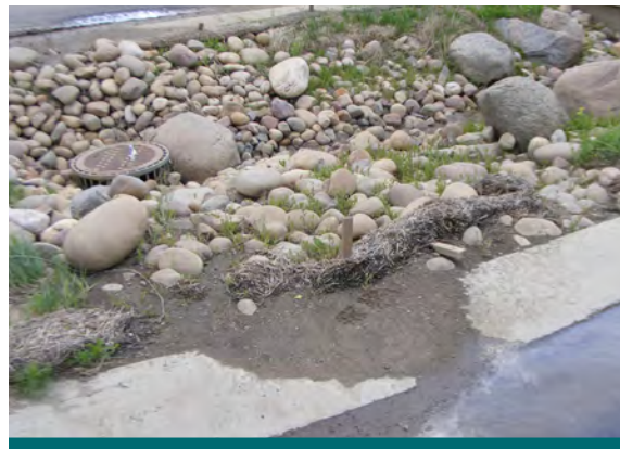
Figure 10.3.1: Failure of sedimentation and erosion controls may cause significant impairments to infiltration practices. In this instance, wait until construction has finished before rehabilitating bioretention area. (Source: Aquafor Beech)
