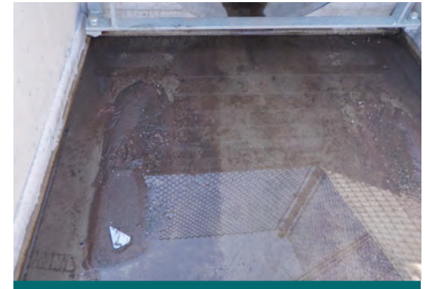
Figure 10.2.4: Along with measuring sediment depth in a proprietary stormwater treatment device, check the outlet structure if accessible. If the OGS is functioning as intended, sedimentation should not be occurring. (Source: Aquafor Beech)
