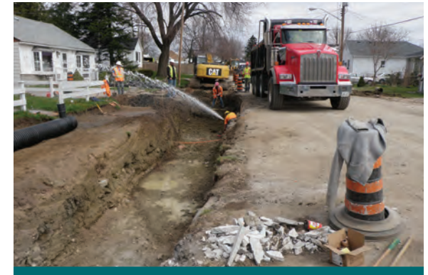
Figure 9.4.2: The costs associated with damage to a pipeline or utility will depend on the type of utility and may include response, repair, environmental impact mitigation measures, and restoration. (Source: Aquafor Beech)
