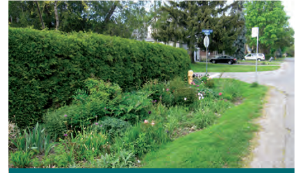
Figure 4.3.4: While many homeowners of this Toronto neighborhood have kept their enhanced swales as grass, a few have turned their swales into gardens that increase stormwater treatment and infiltration. Note that only low growing vegetation was used to avoid encroach on street corner sight lines. (Source: CVC)
