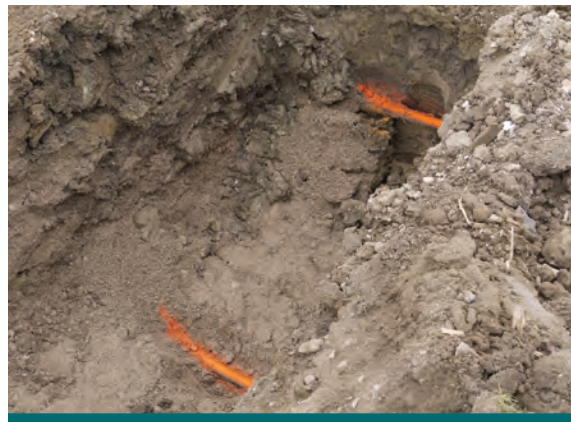
Figure 9.4.1: To prevent damage to pipelines and utilities, daylighting is done prior to excavation with heavy machinery in the vicinity of the utility locate. In this photo utilities are marked with orange paint after being exposed. (Source: Aquafor Beech)
