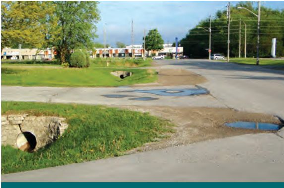
Figure 4.3.14: Local industrial road. (Source: Aquafor Beech)
