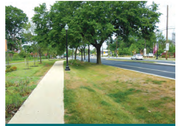
Figure 4.3.19: Enhanced grass swale located between the curb and gutter in Washington, DC. (Source: LID Center)
