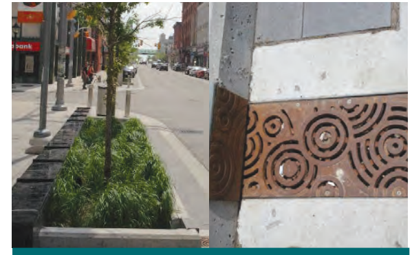
Figure 4.3.31: City of Kitchener incorporated bioretention planters into their main commercial street, King St. The design incorporates seating and trench drains with decorative grating to take runoff from the street. (Source: CVC)
