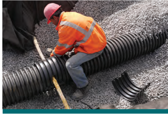
Figure 9.4.6: The next step was placing a piece of perforated pipe on top of the gas line to prevent blockages in the pipe when the trench was filled with clear stone. (Source: Aquafor Beech)
