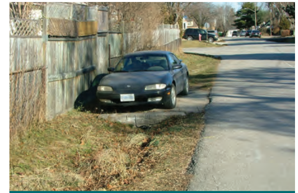
Figure 4.2.3: Encroachments onto the ROW are unlikely to be identified on background materials. In this example, a parking space had been created within the ROW. (Source: Aquafor Beech)
