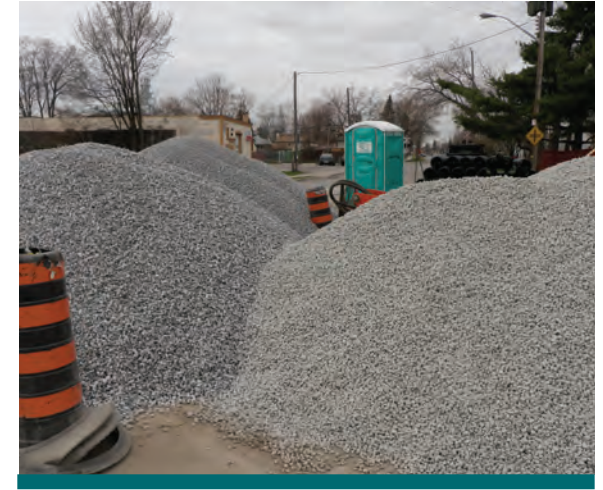
Figure 9.3.2: To the untrained eye both stockpiles of clear stone look similar. An experienced construction supervisor would be able to differentiate the single-washed stone on the right from the double washed on the left. In this case, double washed stone was specified to prevent clogging of the system with stone dust. (Source: Aquafor Beech)
