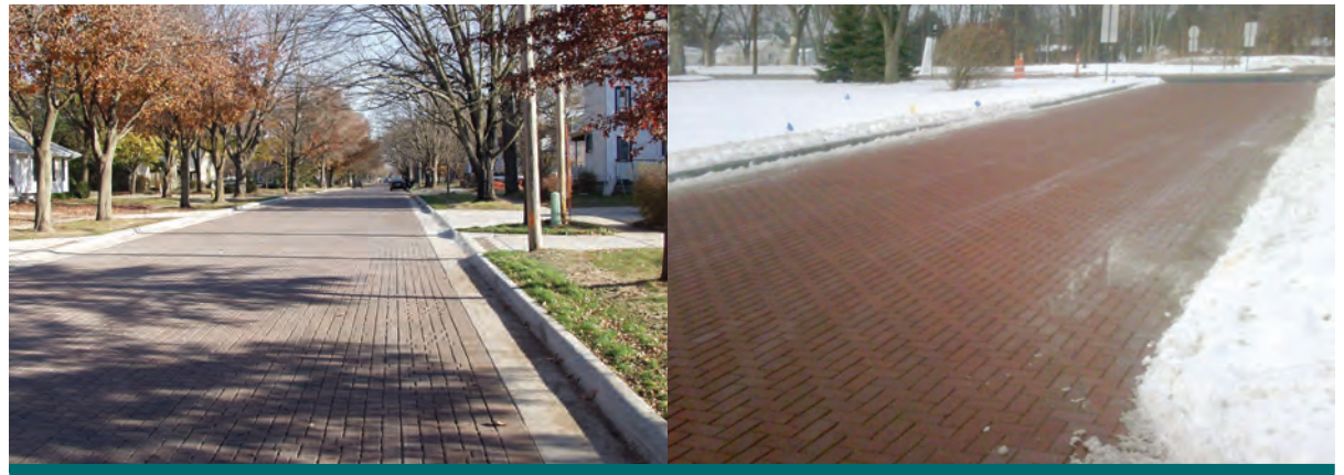
Figure 4.3.7: Permeable pavers used from curb to curb in Charles City, IA (left) and New Albany, OH (right). There are many examples of permeable pavement for the full road within cold climate regions of the US. Snow can be ploughed from permeable pavement as with any other pavement. After ploughing remaining snow can melt immediately into the permeable surface thereby reducing the use of deicers. (Source: ICPI)
