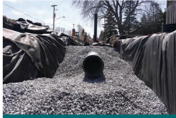
Figure 9.2.1: On-site construction supervisors can verify design elements as they are being built. This perforated pipe will soon be buried. Verifying pipe size, invert elevation, and trench dimensions must occur before the trench is filled. (Source: Aquafor Beech)
