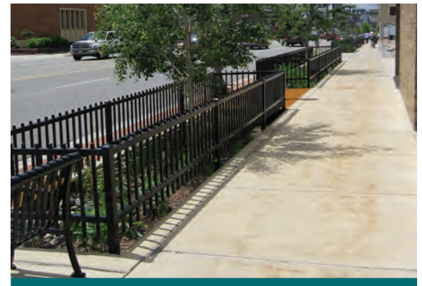
Figure 4.3.32: If grades necessitate a deep bioretention planter, then appropriate fencing should be provided around the planter as was done in this example from Lansing, MI. The Lansing design also incorporated street trees into the planters. (Source: CVC )
