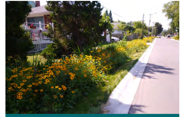
Figure 4.3.8: Boulevard units installed in Mississauga as part of an upgrade from a rural cross section. (Source: CVC)
