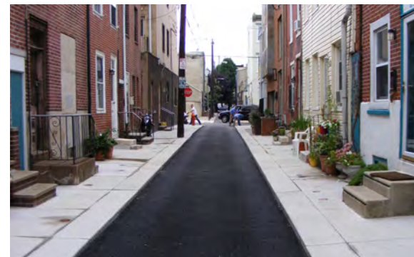
Figure 2.5.1: Porous asphalt and other permeable pavement materials have been used extensively in alleyways and other low-traffic applications in Chicago, IL and Philadelphia, PA (Source: Aquafor Beech)
