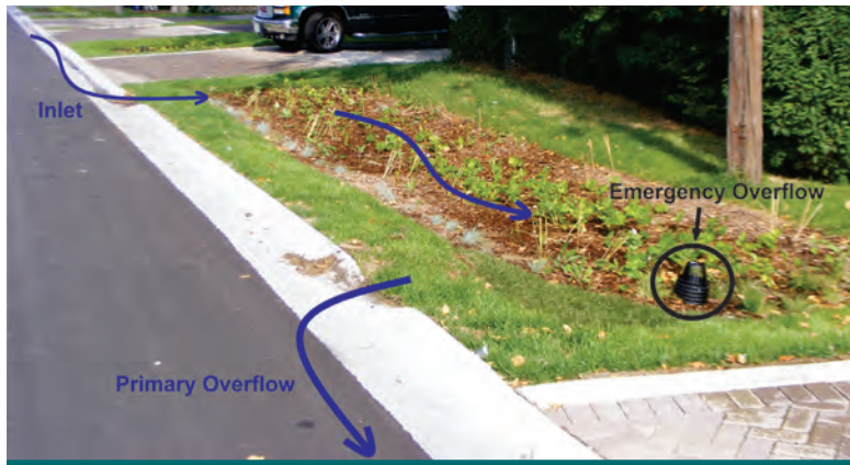
Figure 6.4.8: It is important to maximize the flow path to increase opportunities for filtration and infiltration. The above images of the Lakeview Project show the primary flow path and the location of an emergency overflow. (Source: Aquafor Beech)
