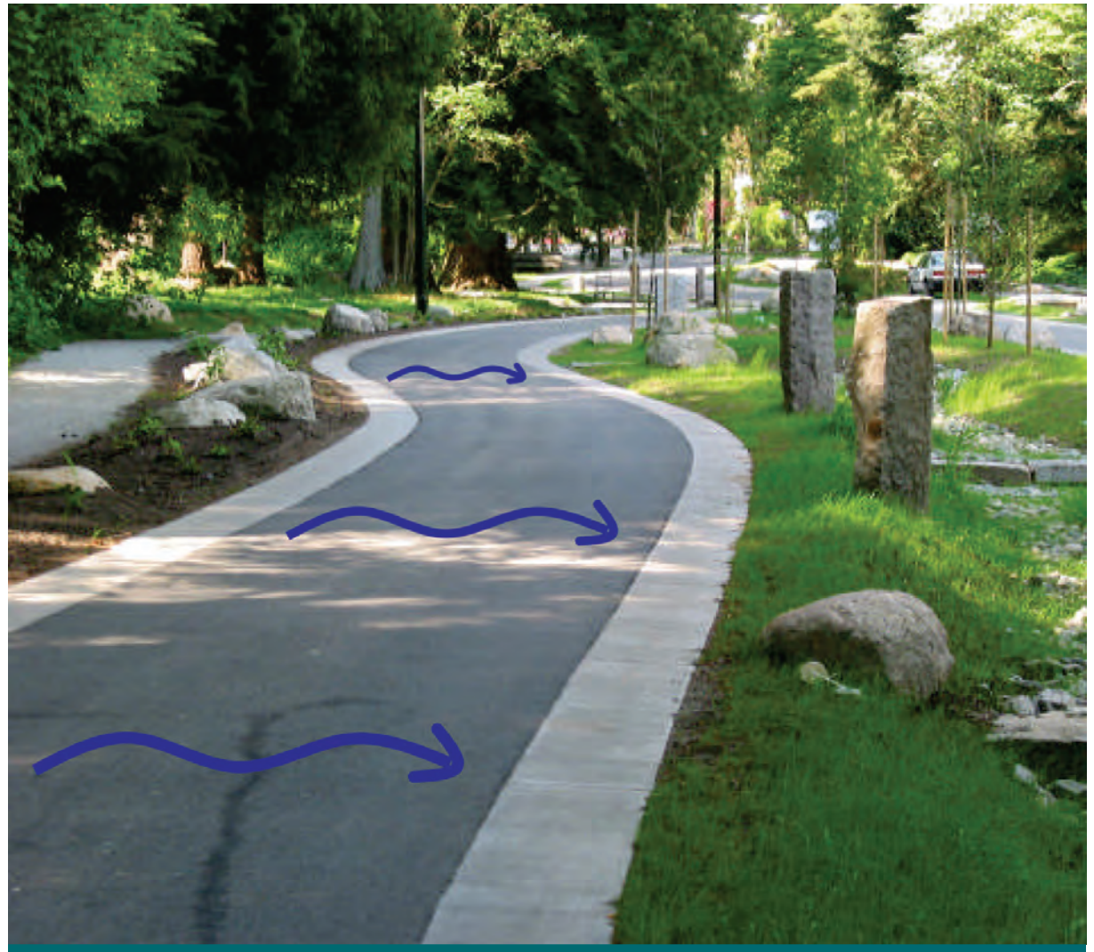
Figure 6.4.1: Flush curbs on both sides of this street allow for drainage from left to the bioswale on the right. (Source: City of Vancouver)
