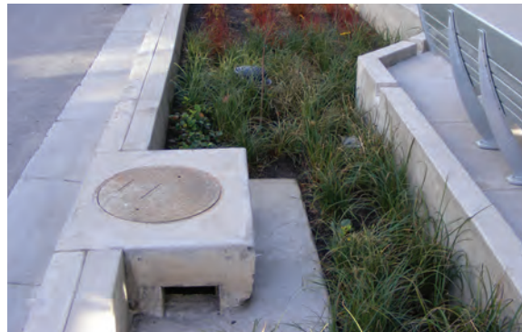
Figure 6.4.5: Inlets and outlets can be incorporated into a manhole by controlling the stage-discharge characteristics with an orifice plate or weir. (Source: Aquafor Beech)
