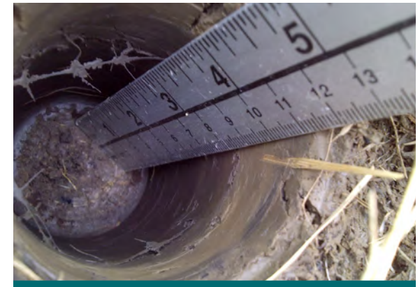
Figure 10.3.2: Coring has indicated that a layer of impermeable clay has clogged this bioretention unit. Major rehabilitation including replacement of the bioretention soil media will be required to allow for filtration and infiltration. (Source: Aquafor Beech)
