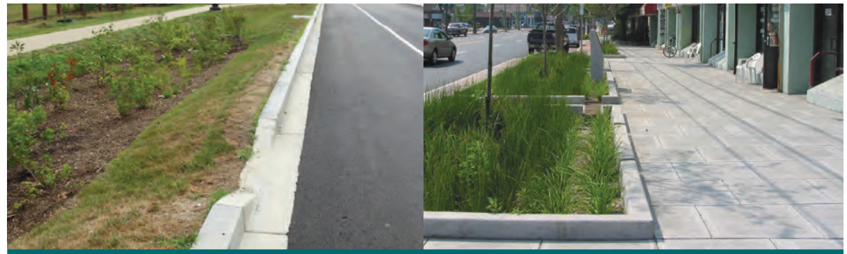
Figure 4.3.23: Boulevard bioretention (left) treating runoff from a minor arterial in Washington, DC. (Source: LID Center). Bioretention planters (right) along a minor arterial in Bridgeport, CT. (Source: Tavella Design Group)
