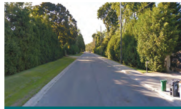
Figure 6.5.3: Low maintenance subsurface practices like perforated pipe systems or enhanced grass swales are best for areas where there is little municipal maintenance and/or high rental rates. In this picture a grass swale is used above a perforated pipe exfiltration system in Toronto, ON. (Source: CVC)
