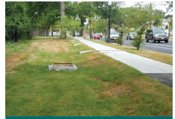
Figure 4.3.20: Grassed bioretention treating road runoff in a wide boulevard space. The grassed bioretention can blend with a corporate property lawn and will be easy for property maintenance staff to maintain with little to no training. (Source: CVC )
