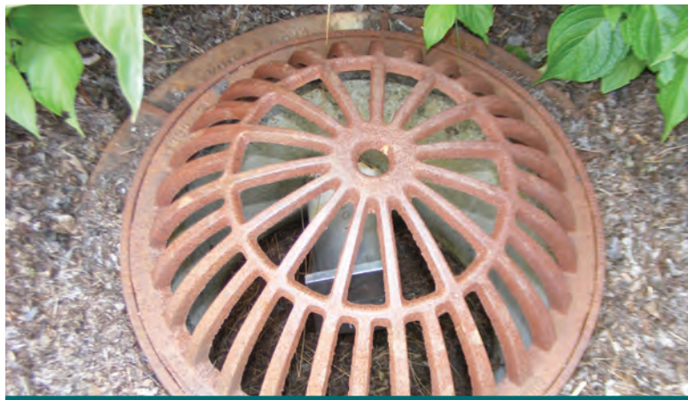
Figure 6.4.9: Properly sized grates can prevent debris from accumulating in storm sewers. Steel grates are recommended because they are more durable than plastic. (Source: Aquafor Beech)
