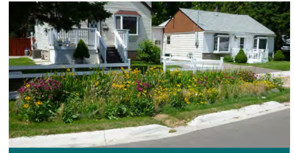
Figure 2.1.7: Boulevard bioretention units are ideally suited for road reconstruction projects upgrading residential streets with a rural cross section to an urban cross-section. This photo shows a home in the Lakeview neighbourhood in Mississauga with a planted boulevard bioretention unit. (Source: CVC)
