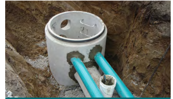
Figure 2.3.1: Perforated pipe systems employ many of the same materials and construction practices as conventional storm sewer pipes, instead using perforated pipes to encourage infiltration during conveyance. (Source: Aquafor Beech)
