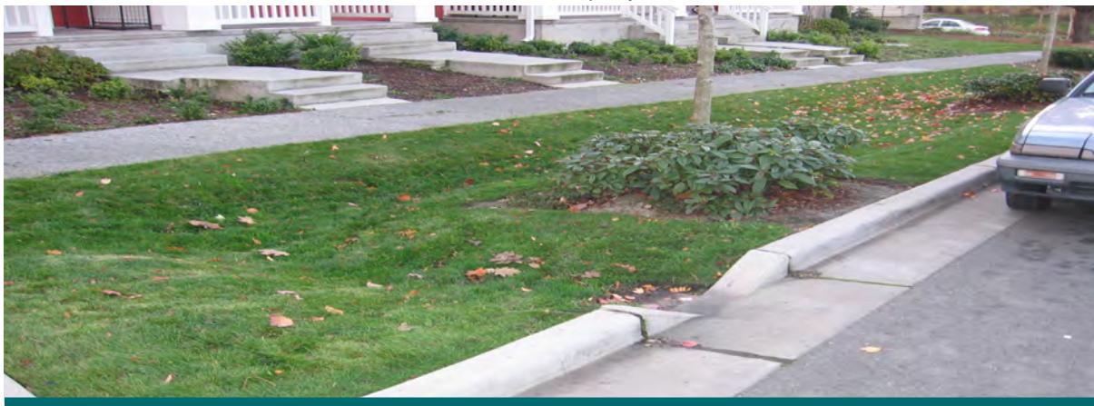
Figure 2.2.1: Enhanced grass swales have been implemented successfully throughout the United States and Canada. (Source: CVC)
