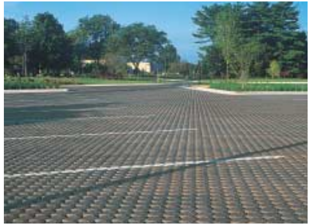
Winter snow-plowing presented no problem for the facility
