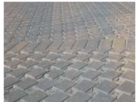
Permeable Ecoloc® and traditional UNI-Anchorlock® pavers were used for the project
