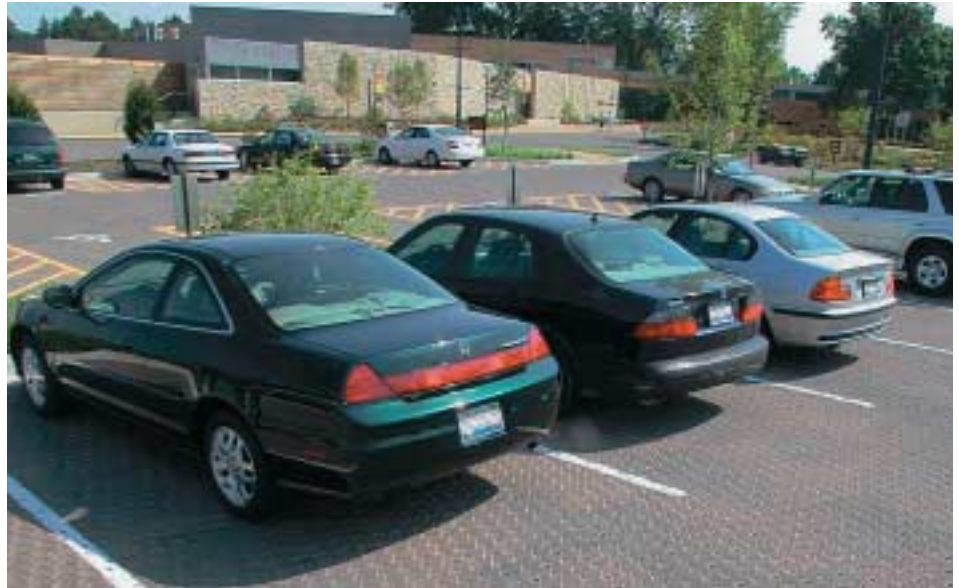
Over 173,000 square feet of Ecoloc® permeable interlocking concrete pavers were used in the Morton Arboretum's 500-car parking lot
