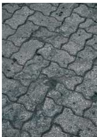
After 9 years of severe impact loads and heavy unpadded tracked dozer traffic, the UNI-Stone® pavers still support current traffic
