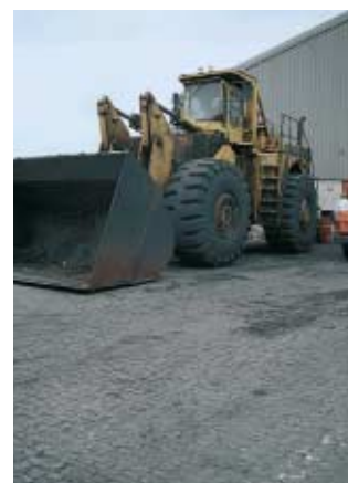
After 9 years of severe impact loads and heavy unpadded tracked dozer traffic, the UNI-Stone® pavers still support current traffic
