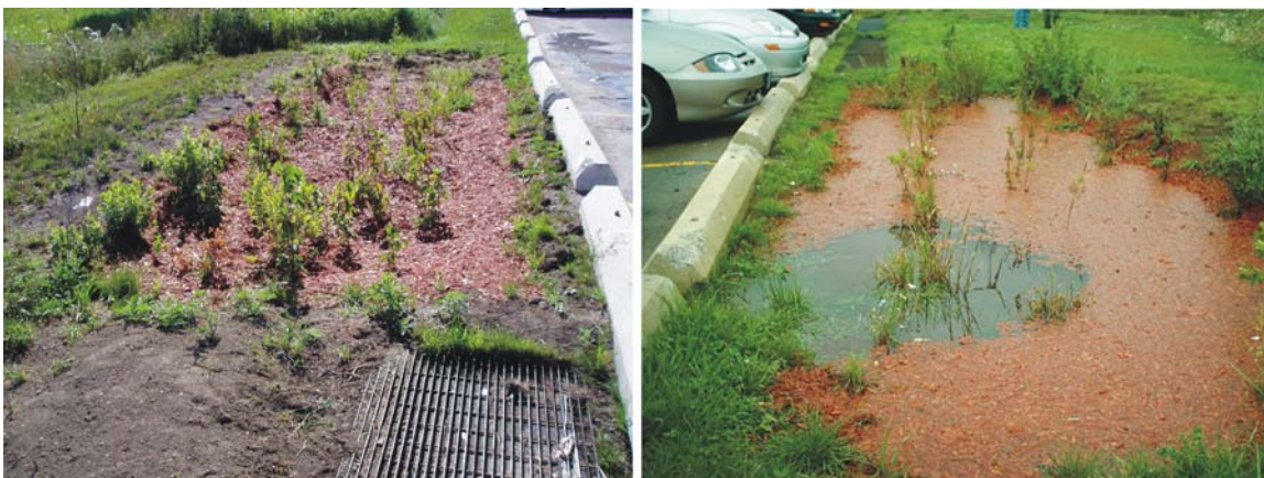
Figure 2 Bioswale during dry weather (left) and wet weather (right).
