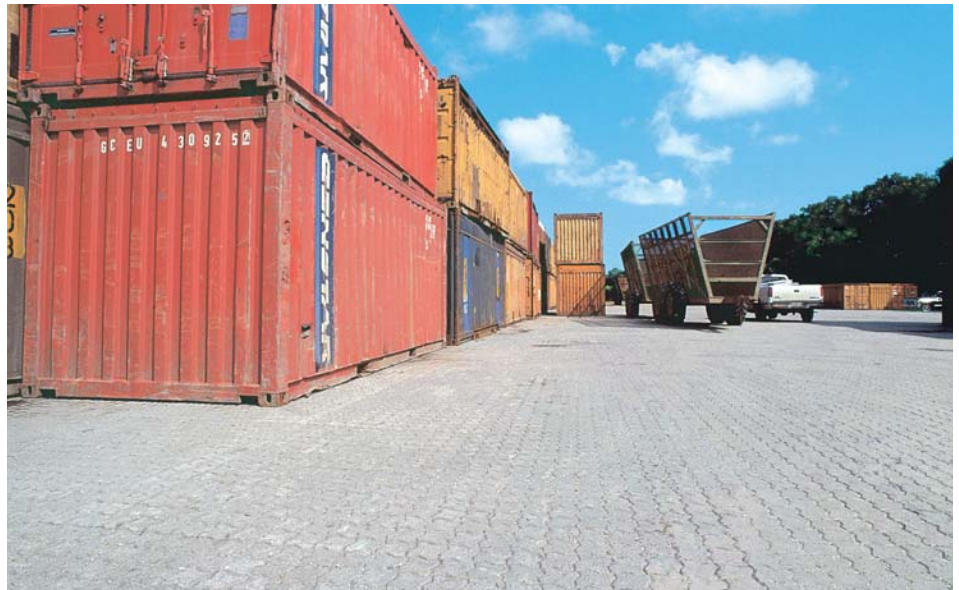
Sterling Sugar features 86,000 sq ft of UNI-Anchorlock ® pavers in their container storage area
