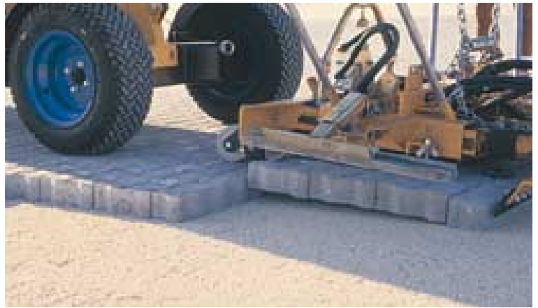
The “anchor-interlocking” shape of UNI-Anchorlock® offers superior resistance to twisting and tipping and is designed for cost-effective mechanical installation
