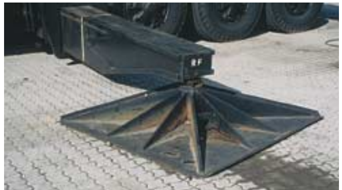
UNI-Anchorlock® pavers are capable of withstanding exceptionally heavy point loads, such as that generated by a 393,000 lb cargo crane
