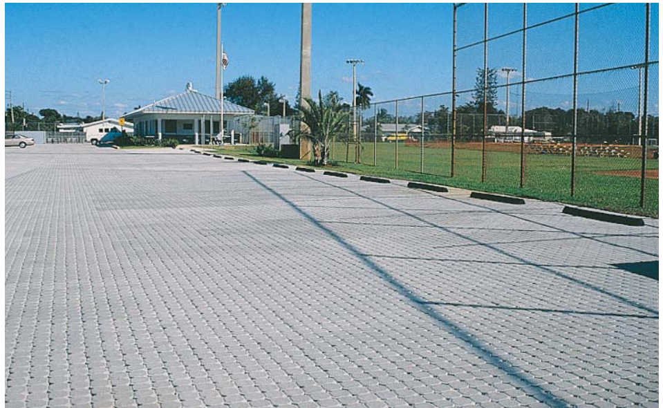
Mickel Field utilizes over 30,000 square feet of permeable UNI Eco-Stone® concrete pavers
