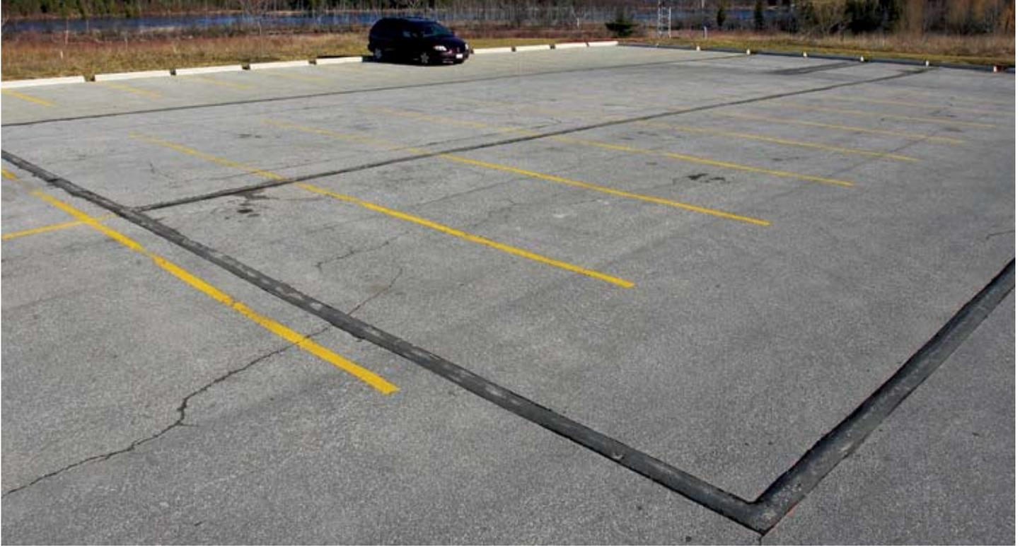
Figure 2. The test area is subdivided in two asphalt areas and one PICP area in the background. The asphalt curbs separate the runoff from each area.
