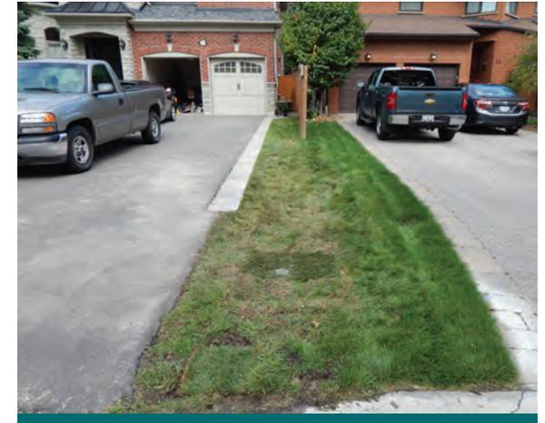
**Figure 3.4.3:** This photo shows the infiltration trench shortly after the turf installation. Instead of turf, plantings could have been incorporated into the design. (Source: Aquafor Beech)
