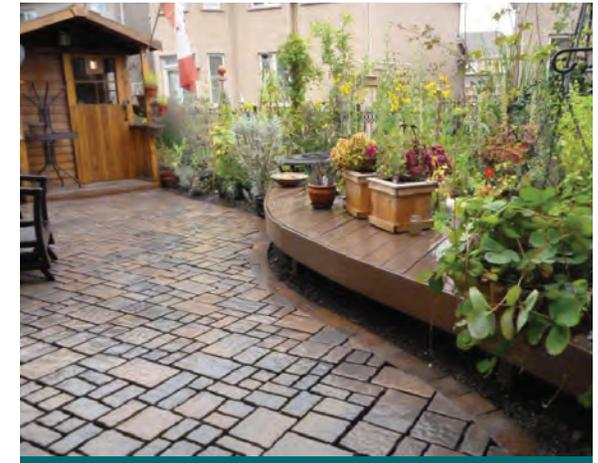
**Figure 3.3.3:** A backyard walkway paved with permeable interlocking pavers (Source: Fern Ridge Landscaping)
