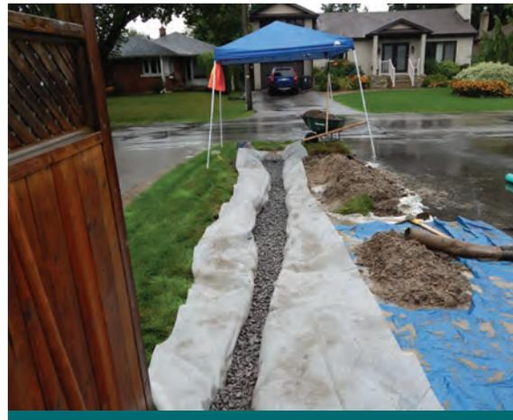
**Figure 3.4.2:** An infiltration trench being installed to improve lot drainage and mitigate basement flooding. (Source: Aquafor Beech)
