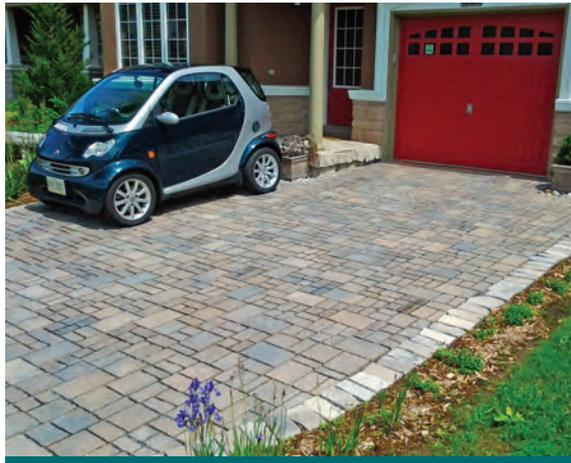
**Figure 3.3.1:** A driveway paved with permeable interlocking pavers. (Source: Fern Ridge Landscaping)
