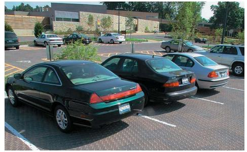
Over 173,000 square feet of Ecoloc<sup>®</sup> permeable interlocking concrete pavers were used in the Morton Arboretum's 500-car parking lot
