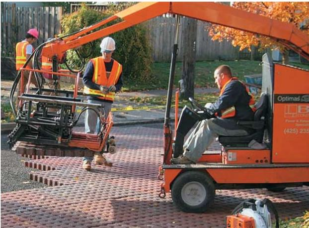
*Mechanized installation allows for fast placement of Ecoloc®*
