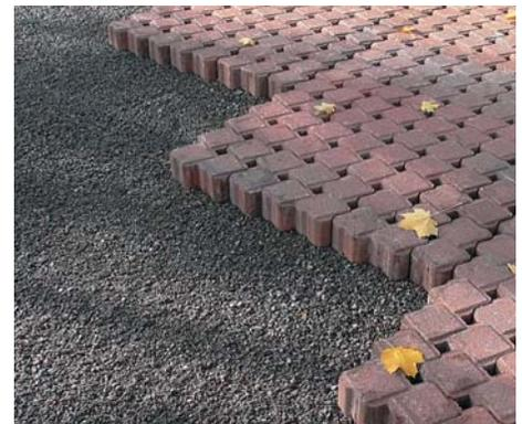
*Ecoloc® pavers were placed on a bedding layer of ODOT 02610.10 open-graded aggregate*
