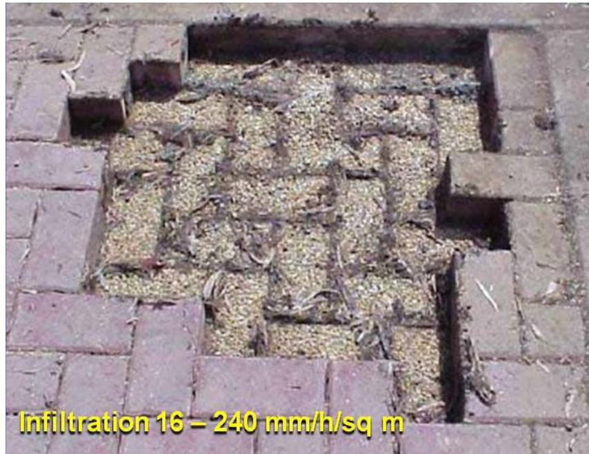
**Figure 2. Excavation at Kirkcaldy Avenue showing penetration of sediment down open joints**
