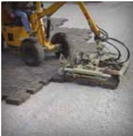
Aggregate base is spread and compacted; pavers are delivered ready to install. After placement of bedding course, joints and/or openings are filled with small aggregate and the pavers are compacted. Joints may be filled mechanically as shown. Mechanical installation speeds construction. Base construction uses locally available materials.
