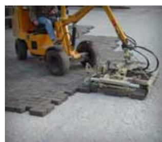
*Mechanical installation equipment accelerates construction; typical 5,000 sf (500 m<sup>2</sup>)/machine/day. After placement, joints and/or openings filled with small aggregate and pavers are compacted.*
