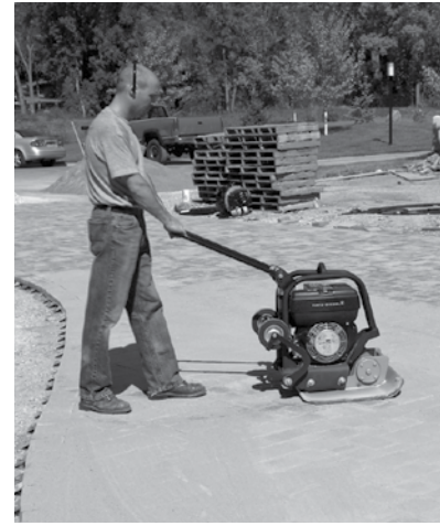
Figure 11. Vibrating sand into the joints.
