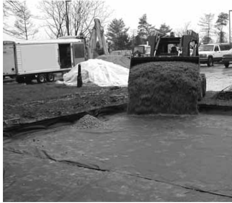
Figure 3. Application of the geotextile under aggregate base.
