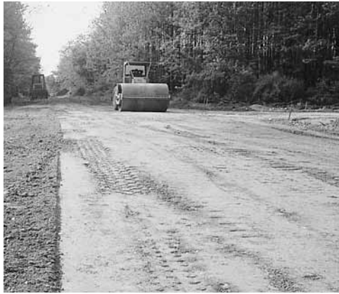
Figure 2. Compacting the soil subgrade.
