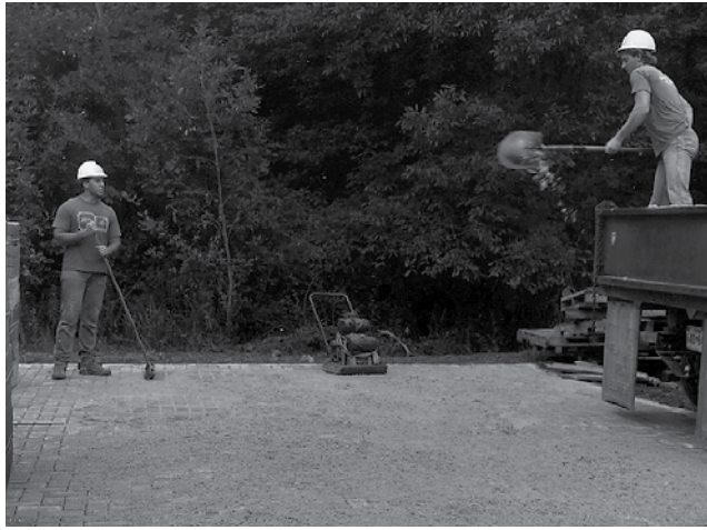
Figure 10. Spreading and sweeping joint sand.
