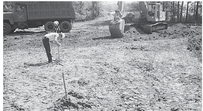
Figure 1. Excavation of the soil subgrade.
