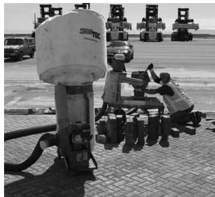
Figure 8. Saw cutting pavers.
