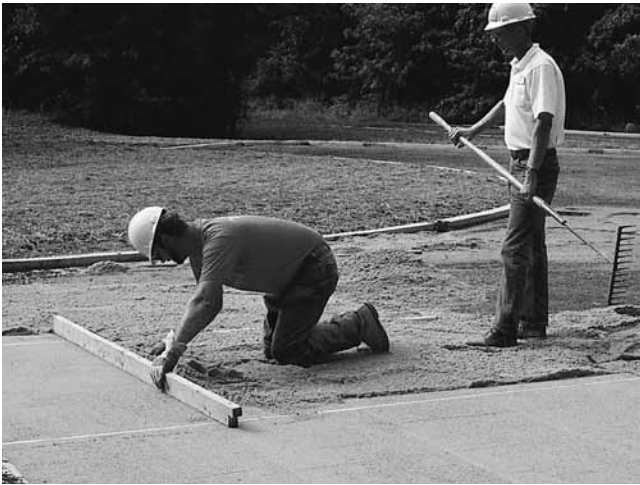
Figure 6. Screeding the bedding sand.
