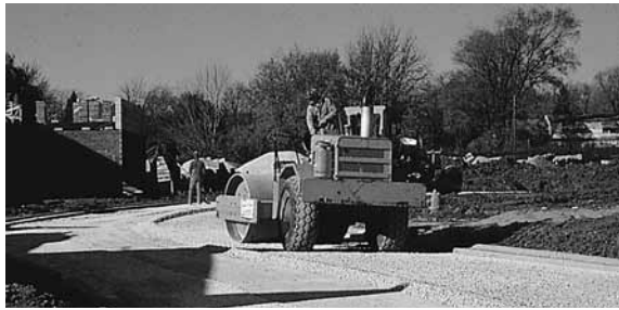
Figure 4. Base compaction with a vibratory roller.
