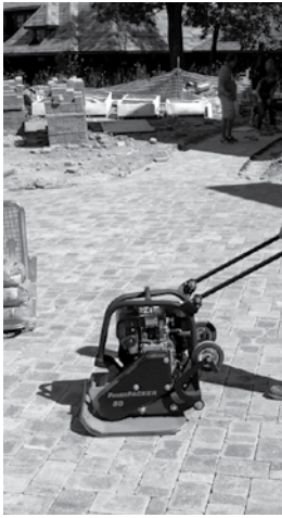
Figure 9. Compacting the pavers and bedding sand.
