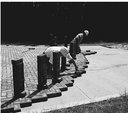
Figure 7. Placing the concrete pavers.
